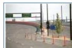
Charles Grimes Bridge
