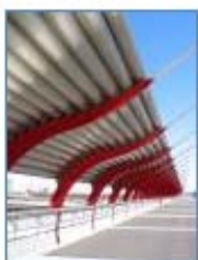
Spencer Street Footbridge
